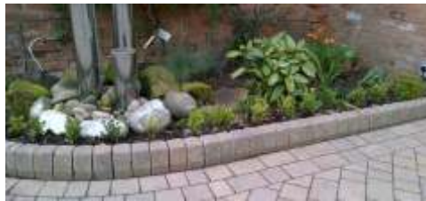
Half batter Low Rise Installation
